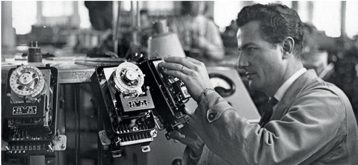
Time switches for automatic staircase lighting systems
